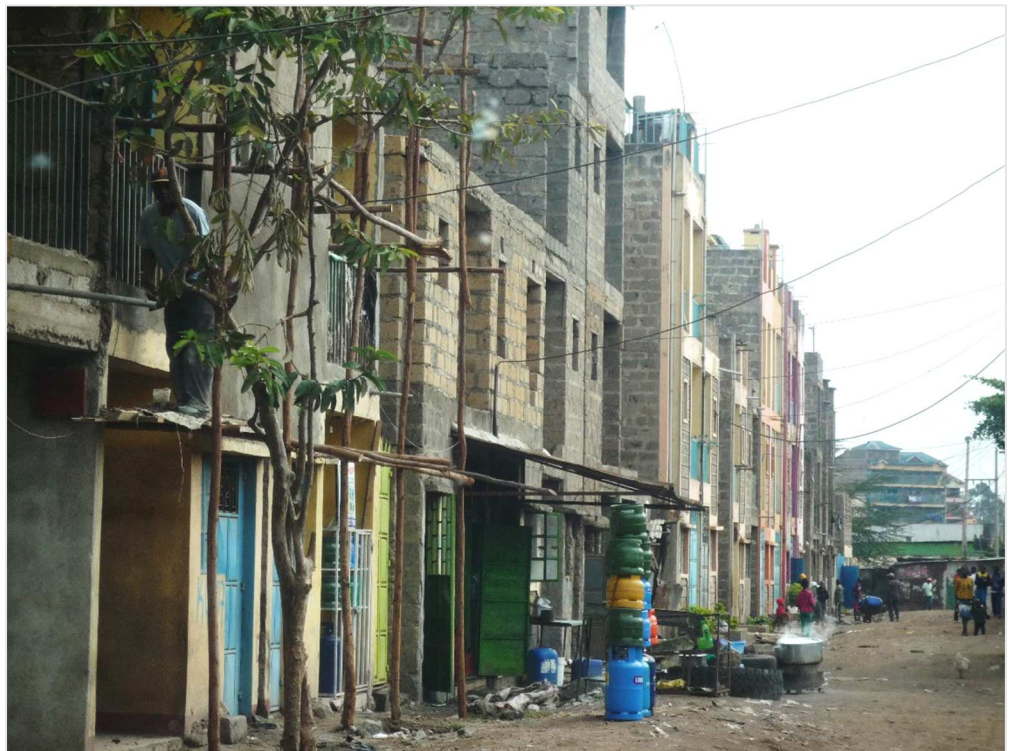
Cooperative housing development in Nairobi (Photo: SUM Consult, 2017)
